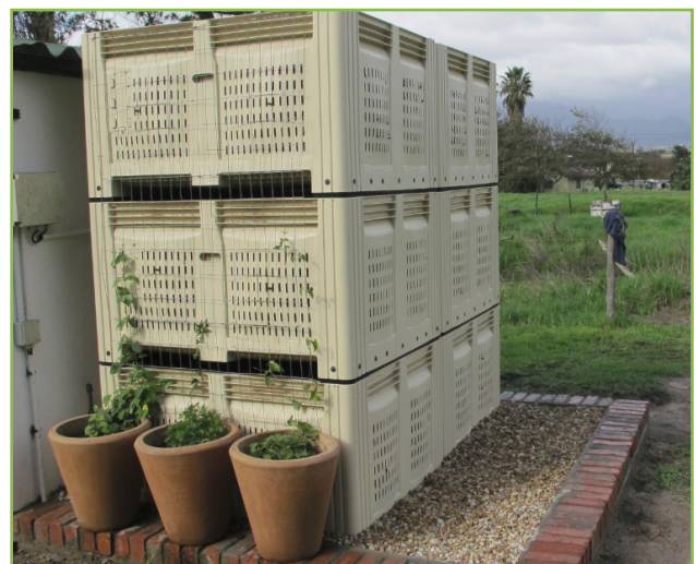
Trickling SOG filter – low energy and highly effective. This unit treats up to 1000 litres per day.
